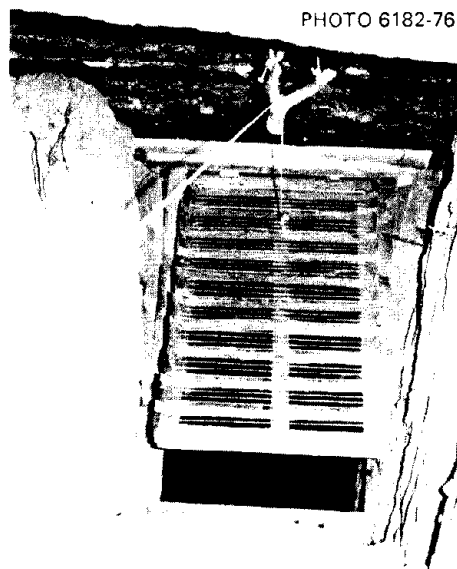
Fig. 17.1. Expedient shelter ventilating pump (a 20 \times 36 in. KAP) in an entry of the Log-Covered Trench Shelter at 53 psi. Tested pre-blast, it pumped 177 cfm through the valves of the two closed blast doors and 412 cfm with the doors open. This entry was demolished by blast effects.
